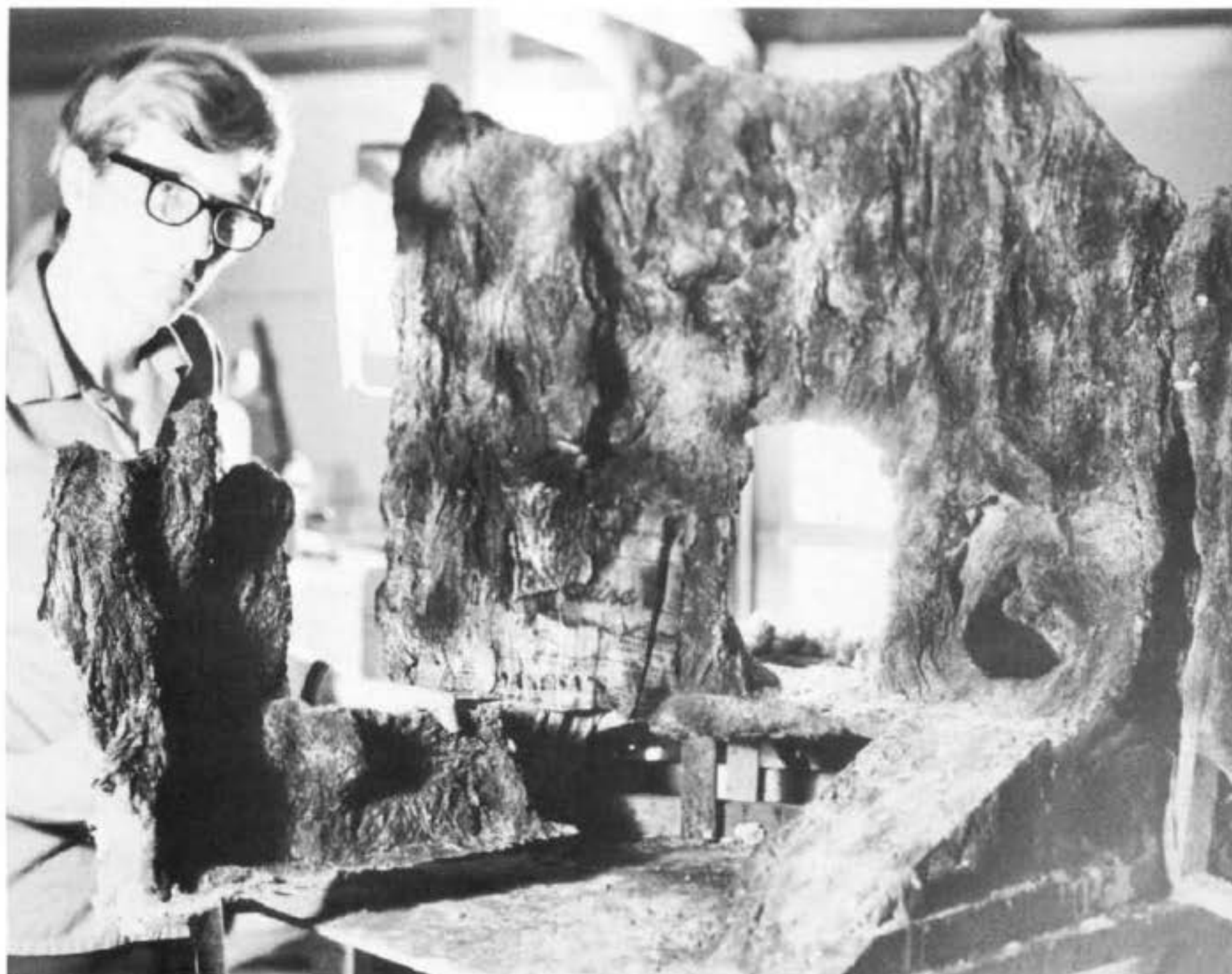
Ernie Farino holds a removable portion of a recently built miniature prehistoric cave set. The cave is made of Hydracol plaster and reinforced, industrial-strength paper toweling.
